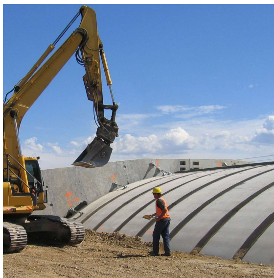
Top: Joints sealed, checking backfill
