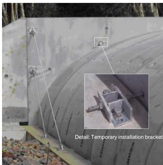
Left: Spandrel secured by tie rods and temporary installation bracket
