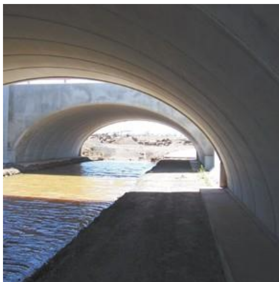
Left: Arch spanning across an existing waterway
