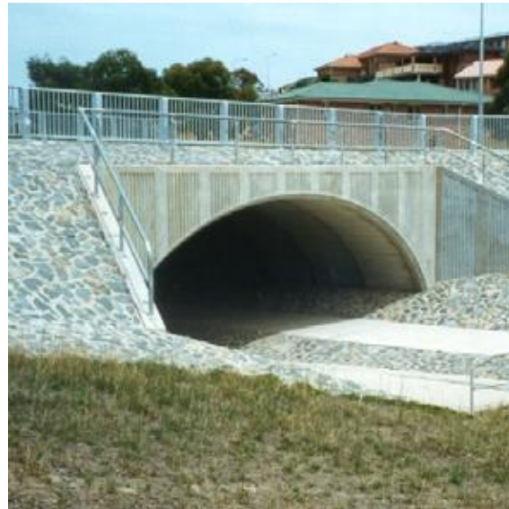
Left: Pedestrian rails attached to the top of spandrel and wingwalls.
