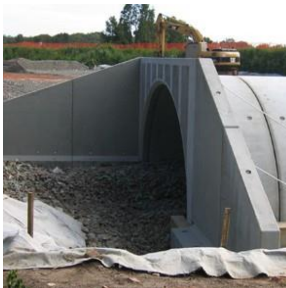
Top: Fully installed wingwalls
