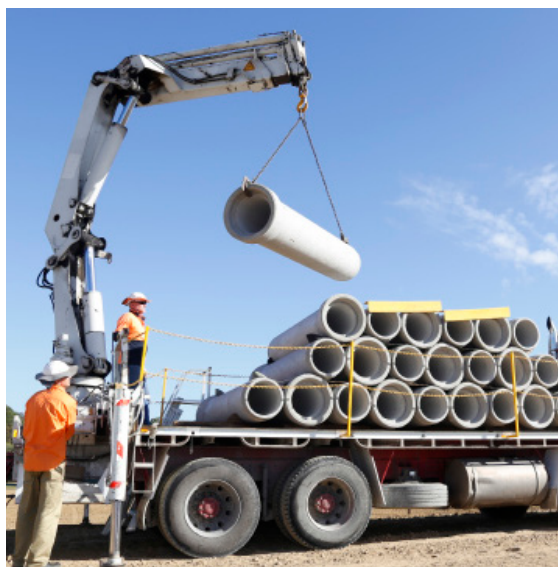
Top: Concrete pipe delivery
