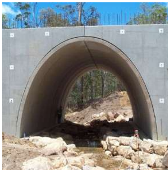
Left: Arch structure spanning a waterway
