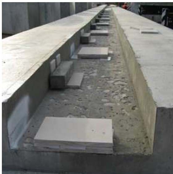
Left: Footings and shim blocks in place
