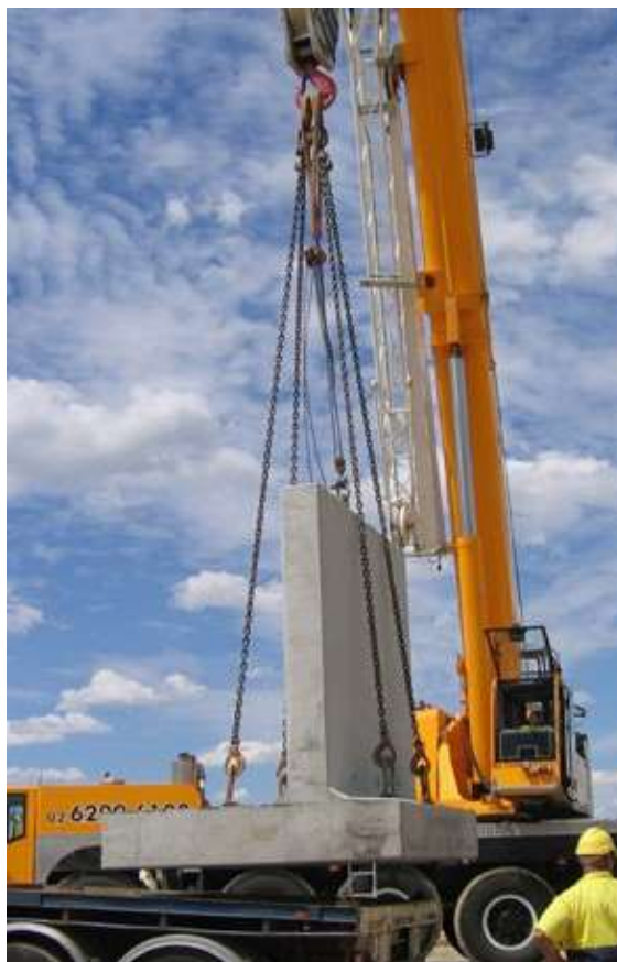
Left: Lifting of wing wall using lifting chains and safety sling
