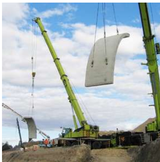
Top: Arch units being lifted from truck
