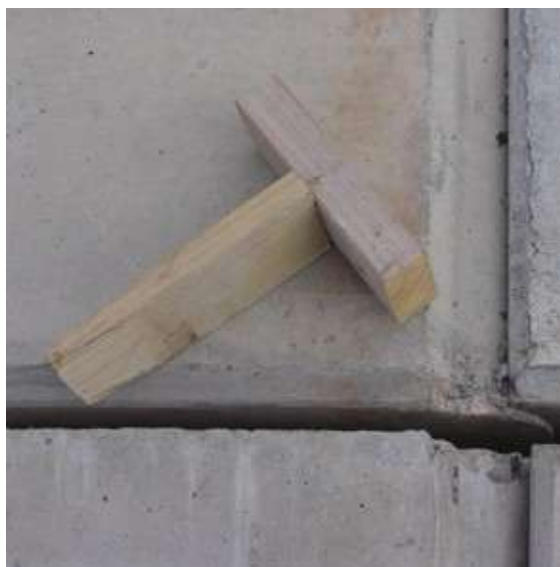
Top: A tee wedge (used to maintain joint gaps)
