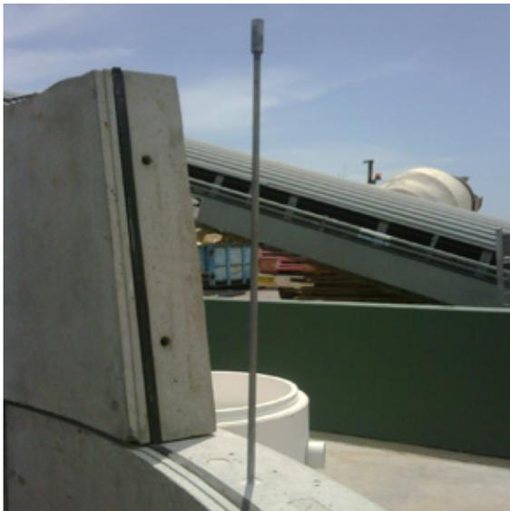
**Figure 12 – Tie rod connection used for caisson installations**
