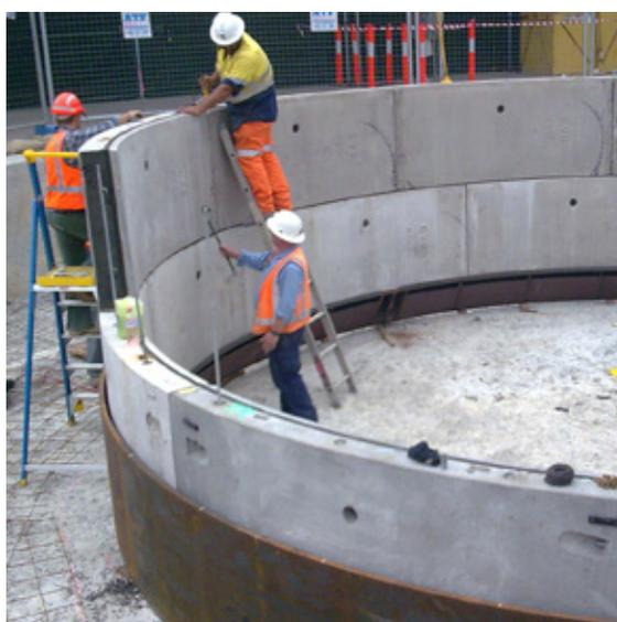
fluid in the annulus above the ring is retained. The choker segments are also designed to bolt the steel cutting edge to the shaft and connect the underpin segment. Refer to combination method on page 11.
