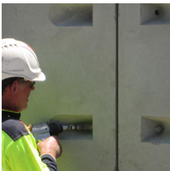
Figure 10 – Curved bolts used for cross joints
