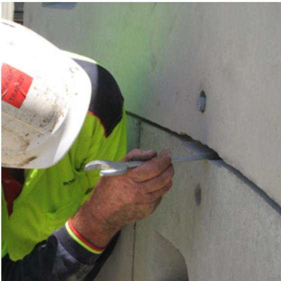
**Figure 13 – Double eye bolt used for underpin installations**
