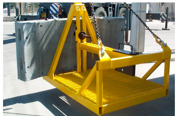
Segment placed into underpinning frame (underpin installations)
