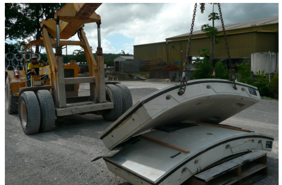
Lifting and tilting the top segment
