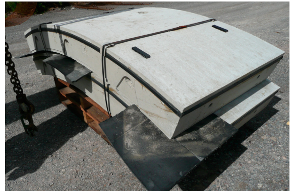
Rubber mats placed between the two segments
