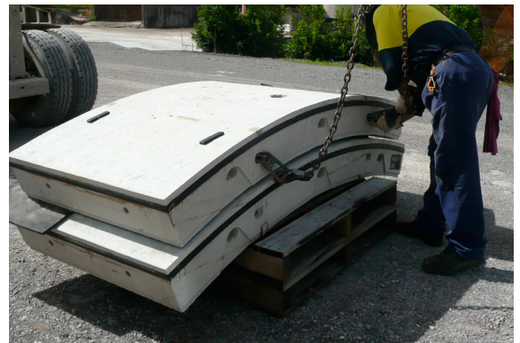
Hooking the clutches into the Swiftlift anchors on the top segment
