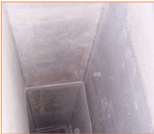
Looking into the AKS lined chamber
