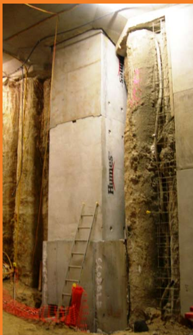
Sewer access shaft inside the busway
